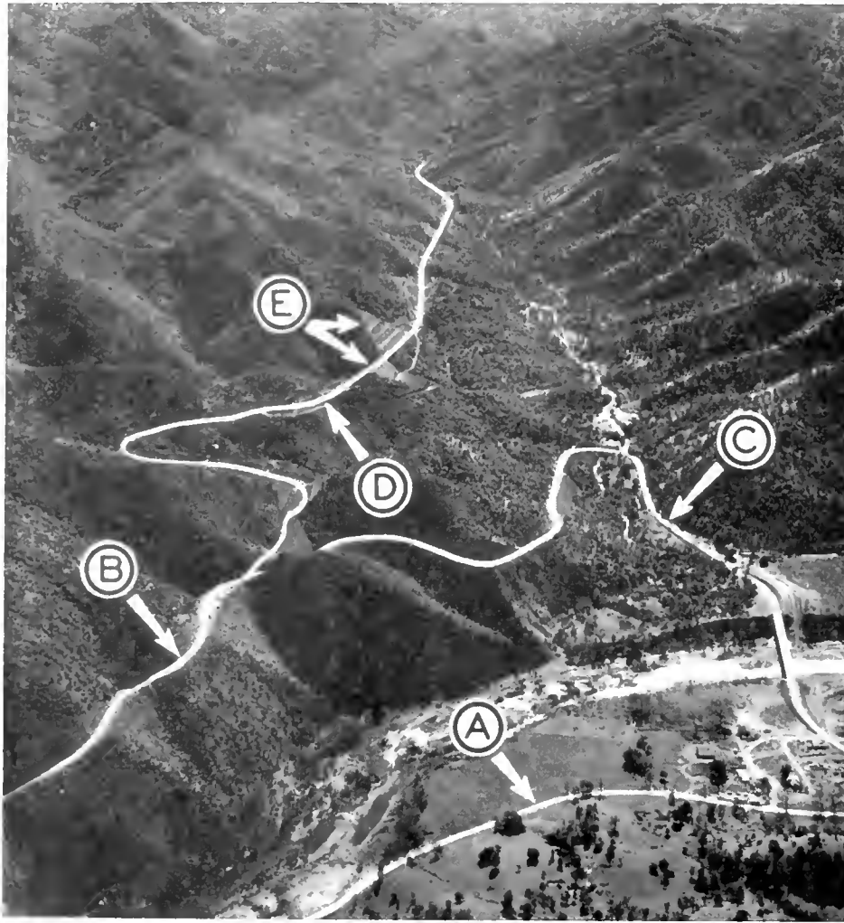
(A) Abandoned State Highway Route 6; (B) Permanent portion, Unit No. 1; (C) Temporary portion, Unit No. 1; (D) Unit No. 2, showing relocated Route 6 winding down into Morkley Canyon; (E) Shows 160-foot fill at Station 118 and 185-foot cut at Station 121
